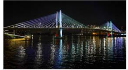
Tillikum Crossing Bridge-don elliot
